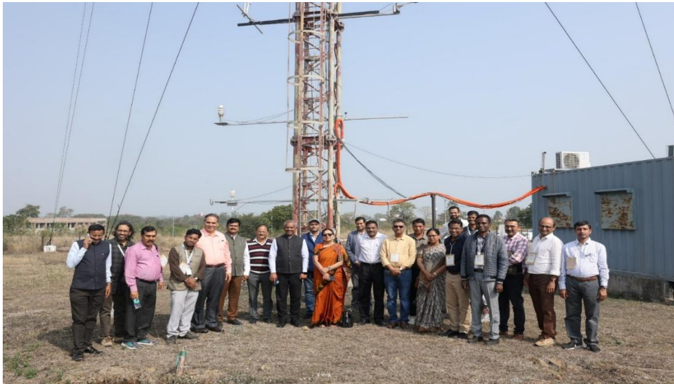
72m Meteorological tower at ART facility
