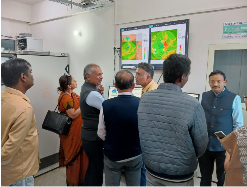
C-band polarimetric radar control room at ART facility
