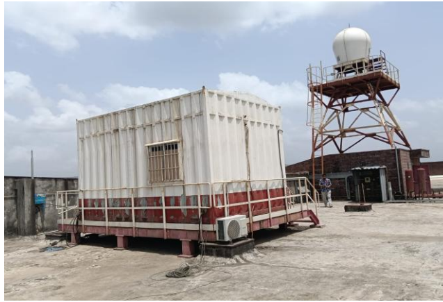
1. Fig. Radar Facility, Amity University, Panvel, Mumbai
