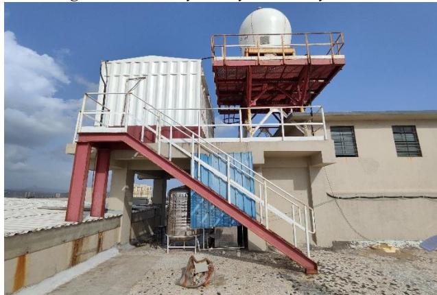
2. Fig. Radar Facility, Vidhyavardhini College of Engineering and Technology (VCET), Vasai-Virar, Mumbai
